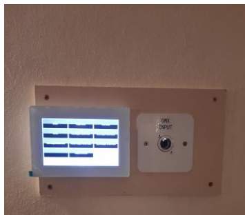
5" touch panel control for day-to-day use with DMX socket for connection of a large lighting control desk
