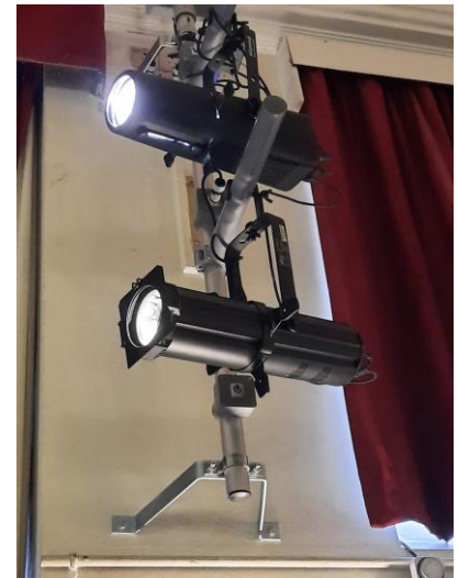
High output LED RGBAL Profile lighting fixtures mounted on one of the two the vertical lighting bars fitted in the main auditorium.
